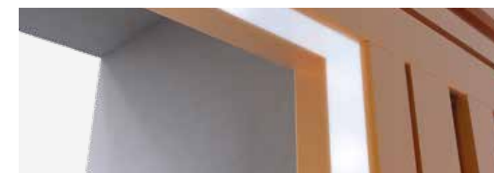
READY FOR INSTALLATION OF GO-LIGHT*
