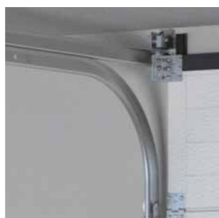
C Double track sliding mechanism
